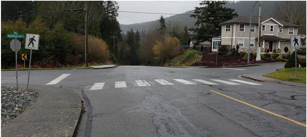
Looking south along Dogwood Drive at Stephenson Street
